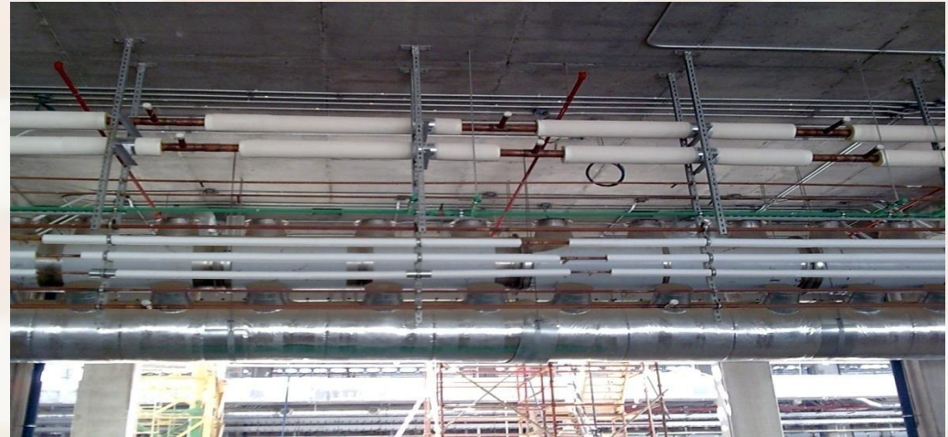
Duct work / copper pipes / C&H. water pipes
