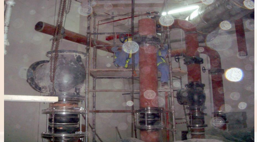
Connections CH.W pipes to pumps
