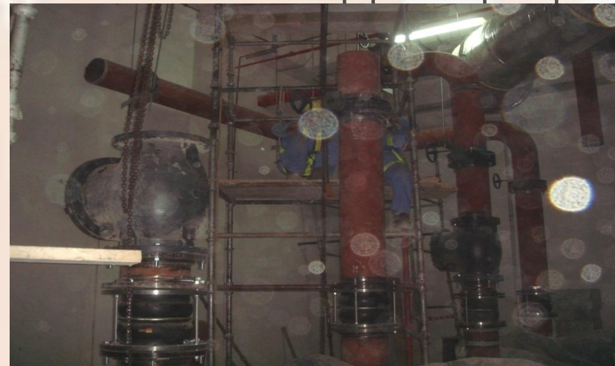
Connections CH.W pipes to pumps
